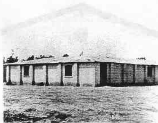
Squadron mess hall - finally completed.
